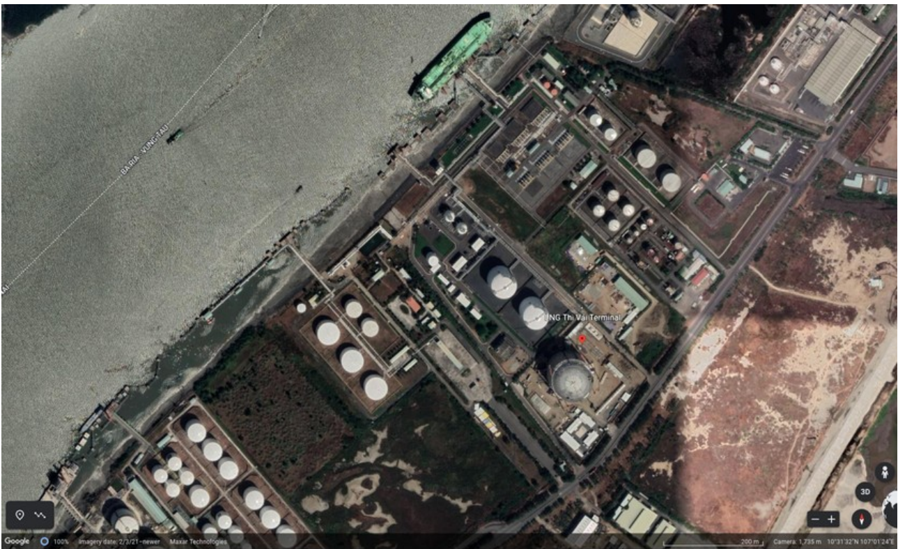
Figure 2: Thi Vai terminal, the first facility to import liquefied natural gas in Vietnam, is due to complete construction in 2022. Source: Google Earth.
