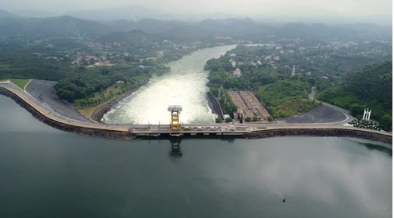
Thac Ba hydroelectric dam at a dangerously high level in 2024. Photo: Chinhphu.vn
