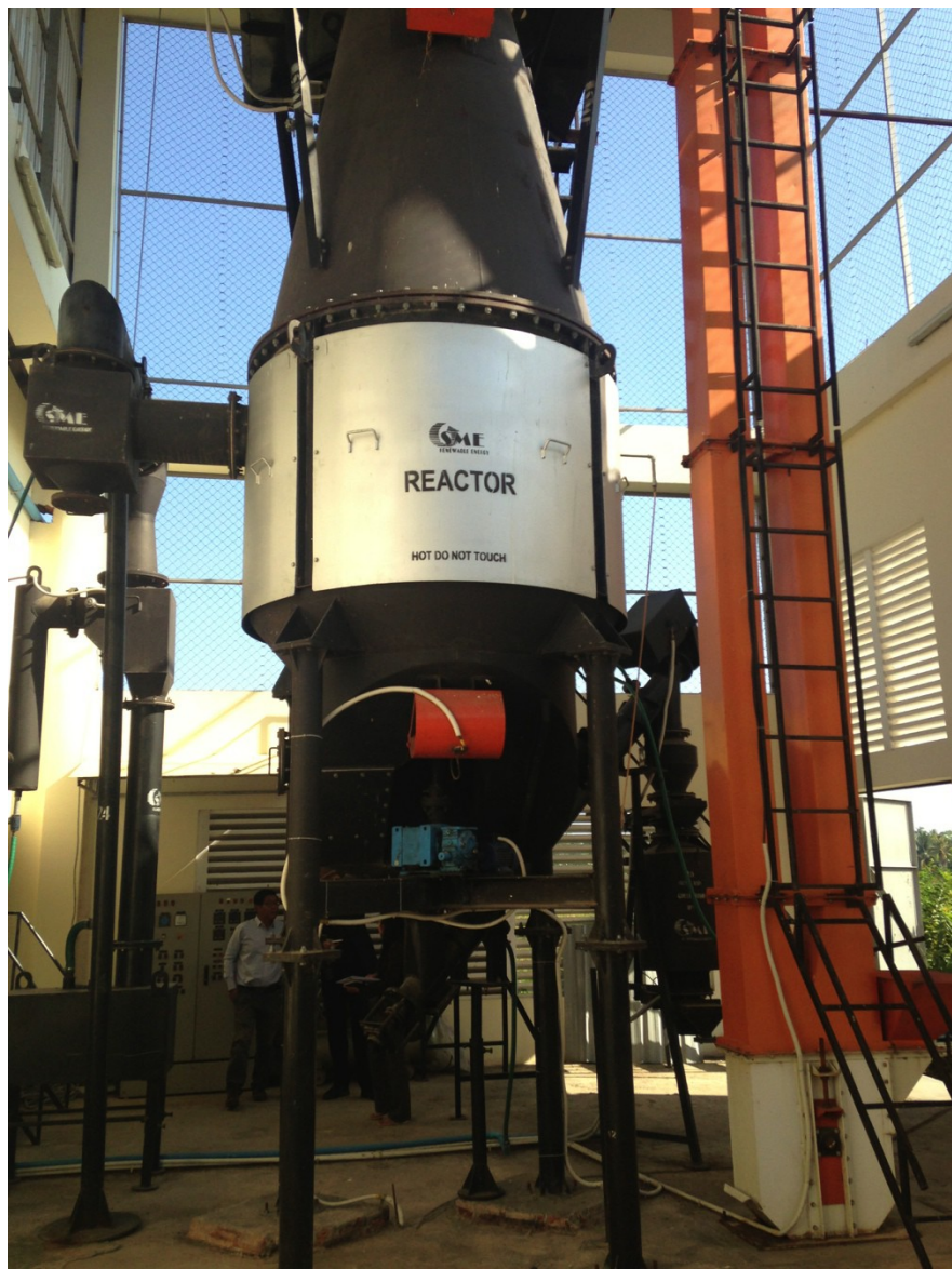
600kW Gasifier at Golden Daun Keo rice mill, Battambang, Cambodia, KH. 2014-12-20
