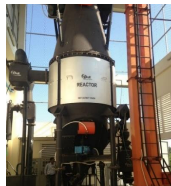
Figure 3: RH gasifier for power generation in Cambodia (Picture taken by author)
